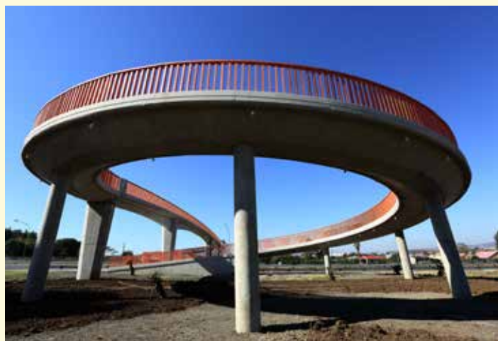
Ladysmith pedestrian bridge
